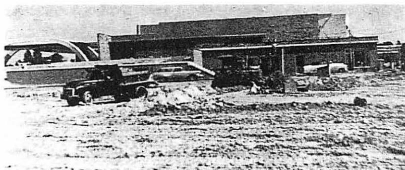
PREPARATION OF SITE AND SUBGRADE
