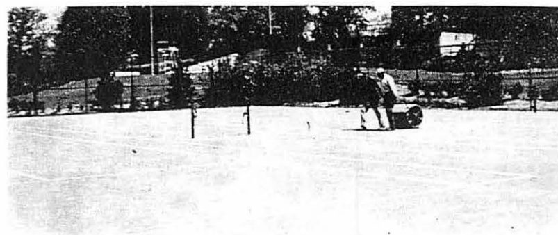
TO FINISH COURT SURFACE
